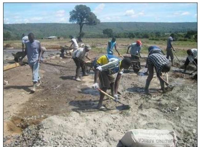
Laying the foundations for the new medical centre - 2013
