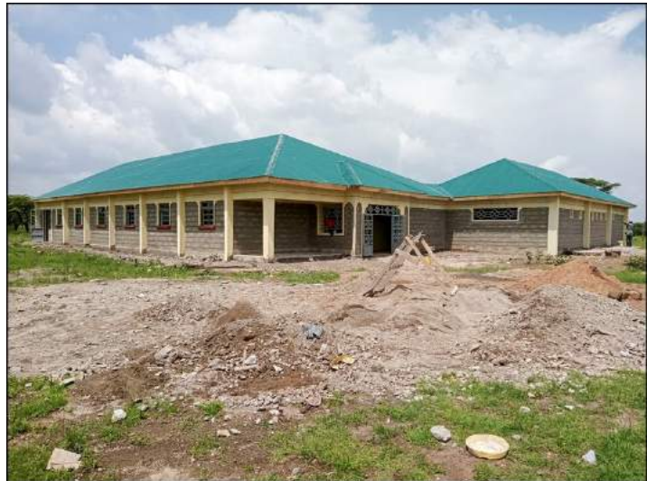
The boys dormitory under construction
